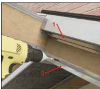
Fitting upper channel 'number 1'
