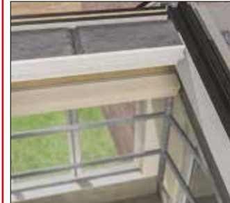
Fitting upper plasterboard trim
