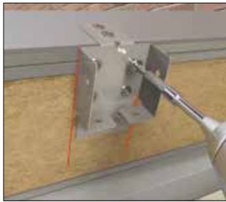
Fixing glazing bar shoes to ridge section
