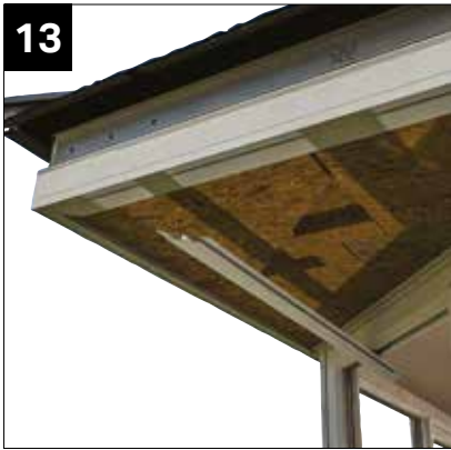
Fit external ship lap cladding edge channel.
