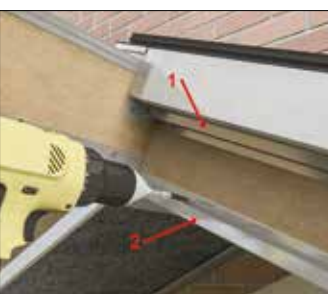
Fitting lower channel 'number 2'
