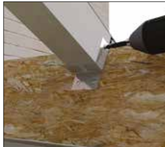
Fixing glazing bar at box beam shoe
