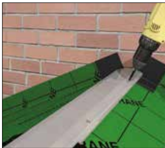
Fixing ridge under capping into tile stop
