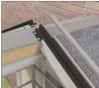
Fixing glazing bar to ridge
