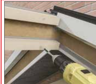
Fitting of the timber ridge battens
