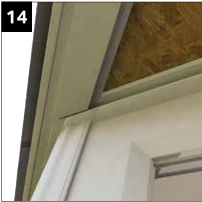
External ship lap cladding edge channel detail.
