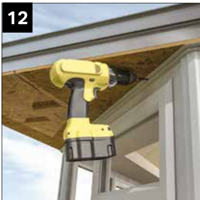
Fit external soffit channeling.
