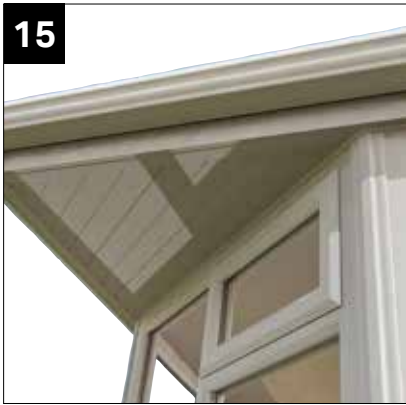
Cut and fit ship lap to suit.
