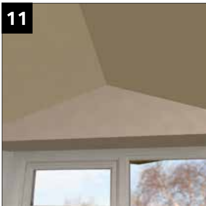
Plasterboard face of gable
