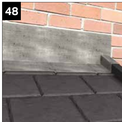
Lead flash to exiting host wall.
