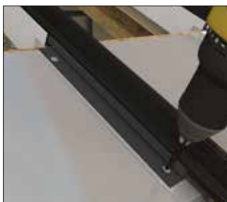
Fixing glazing bar to box beam external face
