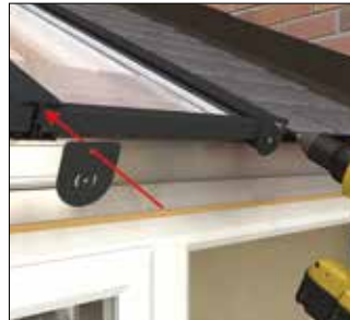
Fixing glazing bar end caps
