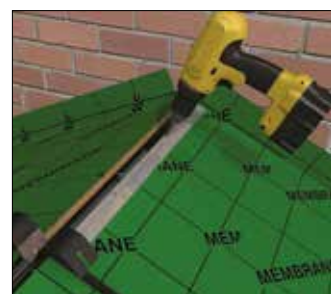
Fixing tile stop aluminium
