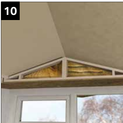
Insulate void with mineral wool.
